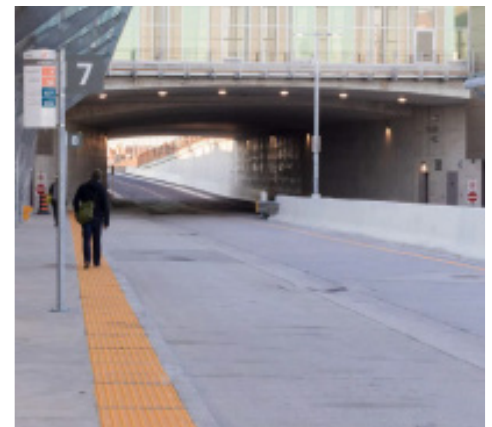
Quick access to Renforth BRT Station
